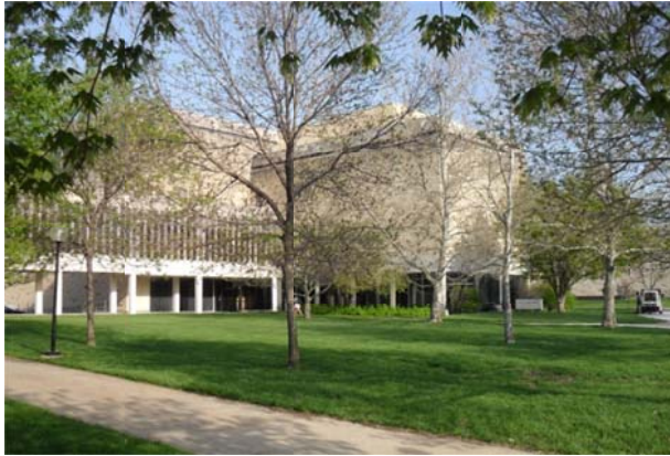
Trotter Hall from the southeast.
